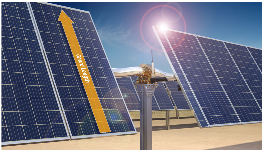
FIGURE 3: Example of chord length, depicted by the orange line.
